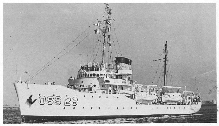
THE MODERN EXPLORER, KNOWN AS OCEANOGRAPHIC SURVEY SHIP OSS 28, IS A 220-FOOT, 1900-TON VESSEL, BUILT IN SEATTLE IN 1940. PRIOR TO CHANGING ITS HOME PORT FROM SEATTLE TO NORFOLK IN THE EARLY PART OF 1960, THE SHIP WAS ENGAGED ON SURVEYS AND OCEANOGRAPHIC WORK IN ALASKAN WATERS. THE SHIP HAS PERFORMED SIMILAR WORK ON THE EAST COAST SINCE THEN. HER RECENT CRUISE, IN WHICH THE SHIP PLAYED AN IMPORTANT ROLE IN EQUALANT I OF THE TRO-PICAL ATLANTIC INVESTIGATIONS, HIGHLIGHTS AN ILLUSTRIOUS CAREER.
